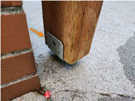
Post Bases not fully fastened
