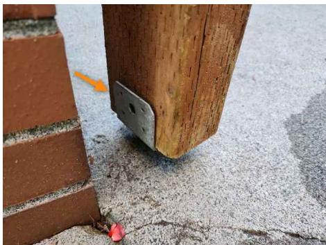
Post Bases not fully fastened
