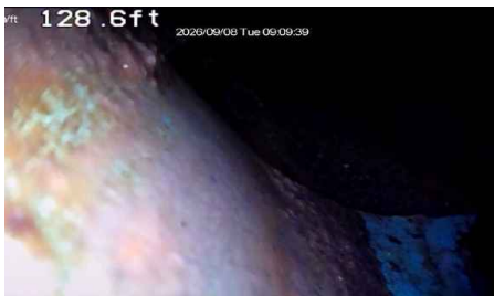
SDR35 to Concrete Main
