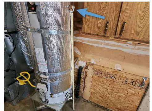
TPR appears to drain to garage slab
